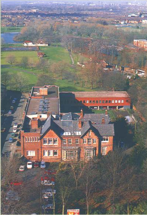
Usdaw Central Office, 'Oakley', 188 Wilmslow Road, Fallowfield, Manchester M14 6LJ.
